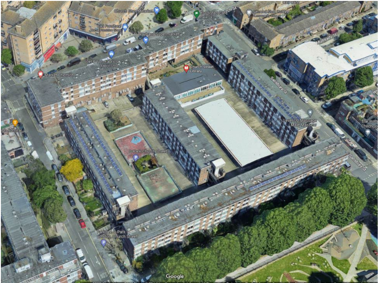
Aerial View of Site B
