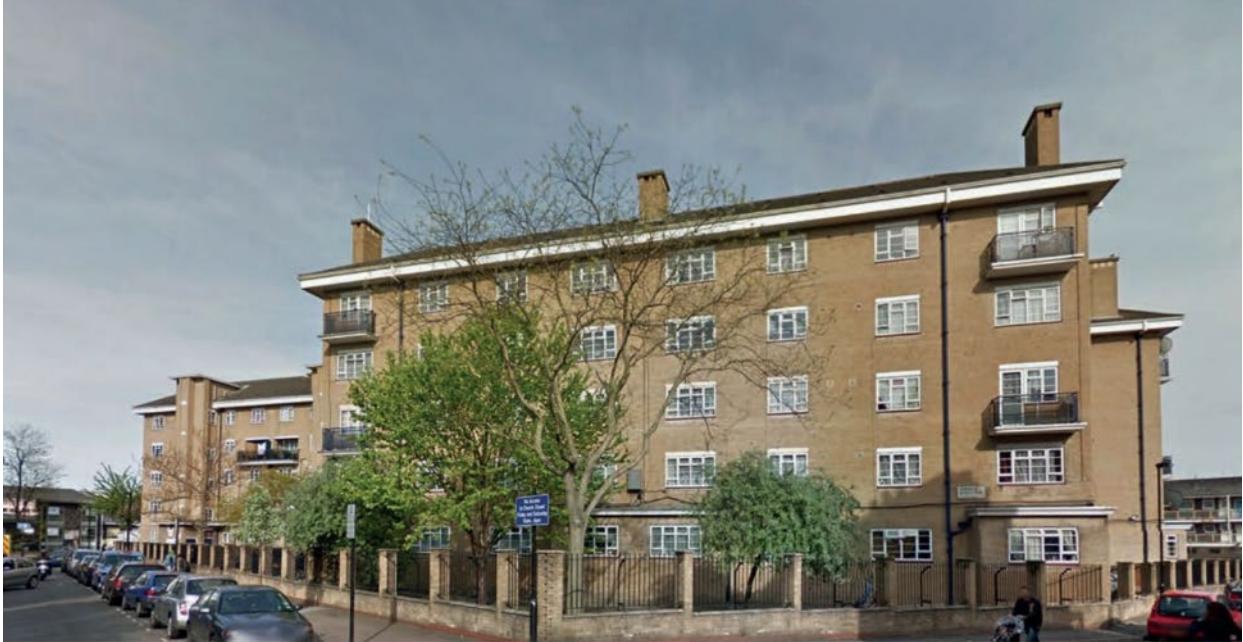
Mole House – Corner of Boscobel and Venables Street (Site C)
