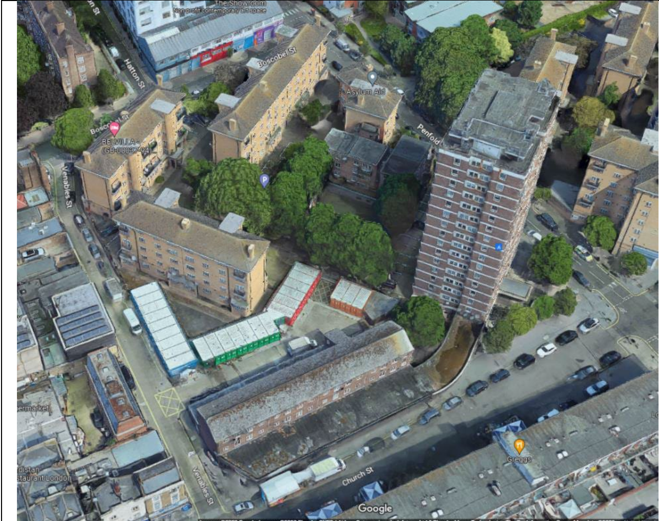
Aerial View of Site C (Kennet House on right is excluded)
